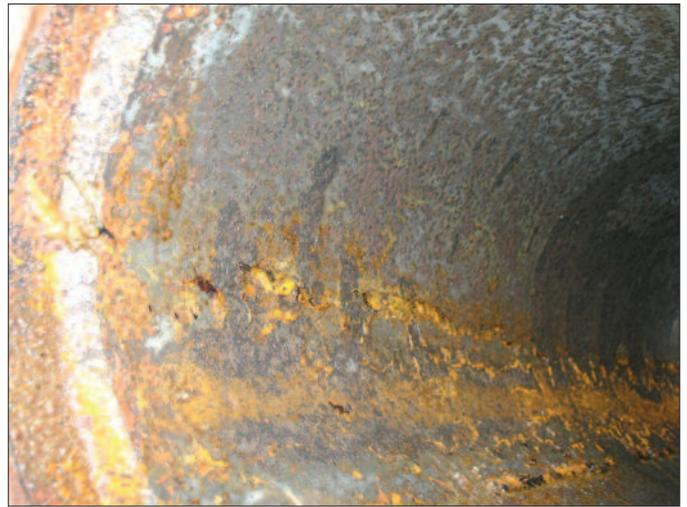
Corrosion pits associated with microbially influenced corrosion.
